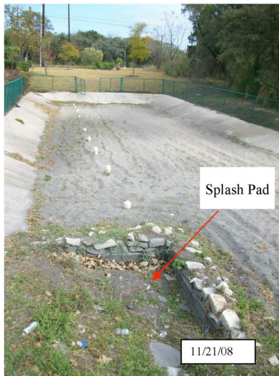
While inspecting the basin the inspector found heavy accumulation of sediment, debris, and vegetation within the splash pad.
