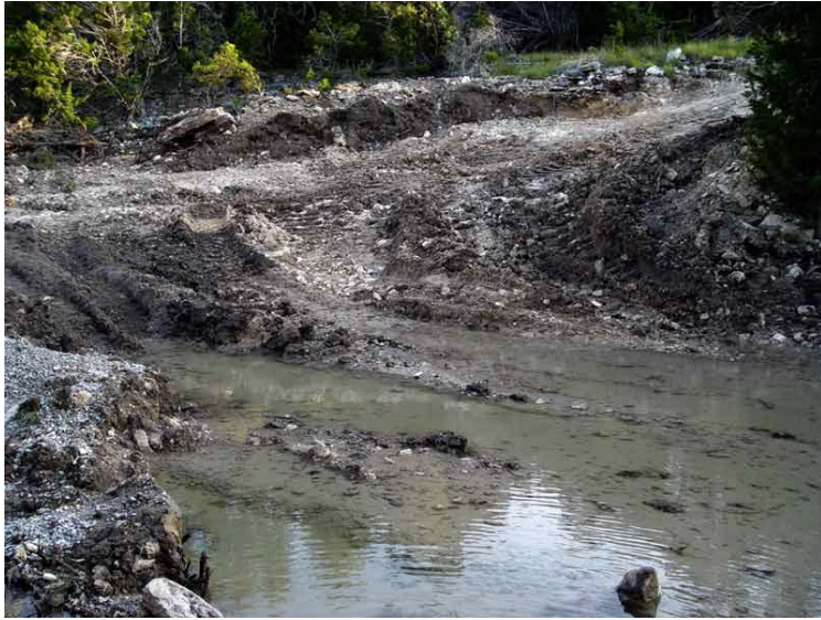
Road cut along Hamilton Creek after rainfall
