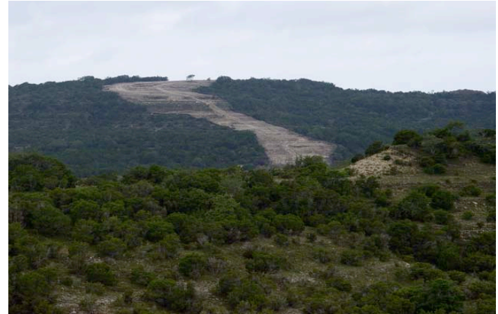
Road cut for land development in Hamilton Creek basin began June, 2007
