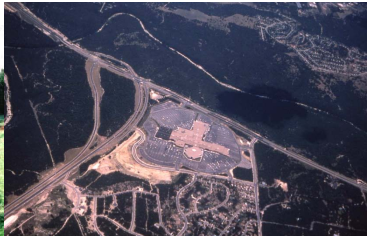
Sand filter – Barton Creek Mall
