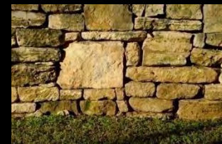
Dry stack stone wall
