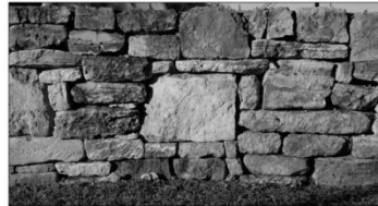
5 SMOKEHOUSE DRYSTACK WALL PHOTO NOT TO SCALE
