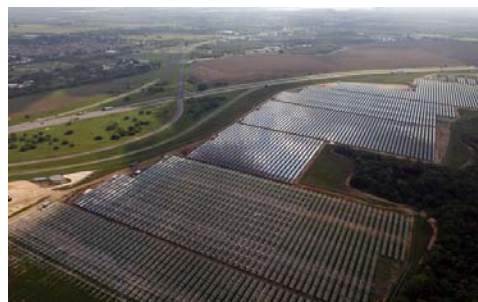
The 14 Megawatt Blue Wing solar facility on San Antonio’s Southeast Side has 214,500 panels on 140 acres making it the largest solar facility in Texas. LISA KRANTZ/lkrantz@express-news.net
