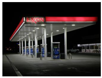
Recessed canopy lights and directed area lighting recently installed at the Blanco Stripes facility provide a safe and attractive environment for customers while protecting Blanco's view of the stars by preventing light from shining up into the nighttime sky.
