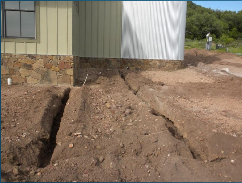
Trenches for piping
