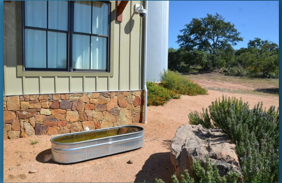
Gutter to underground pipes
