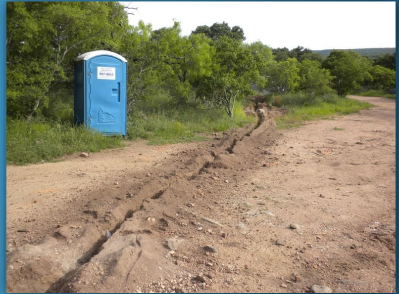
Gravity feed to storage tank
