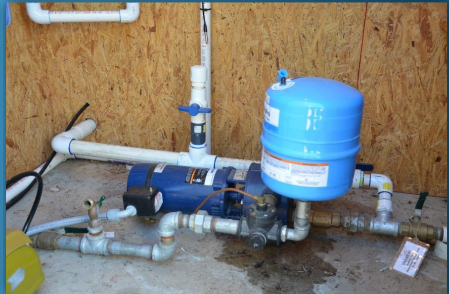
Pump and pressure tank
