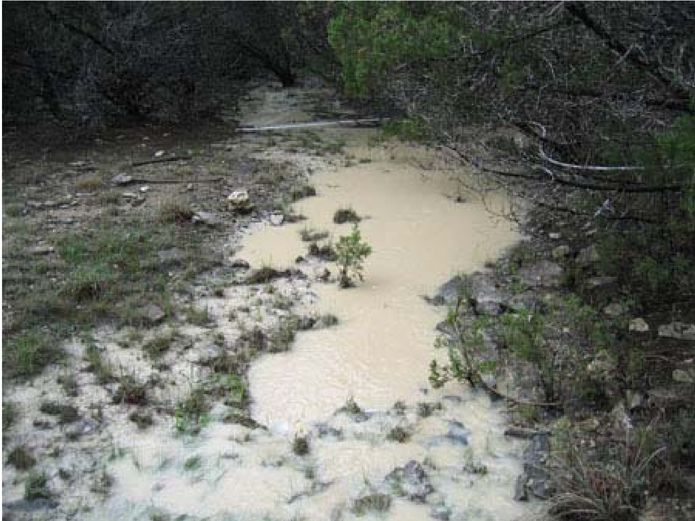
April 2007 photograph of sediment-saturated runoff from the AMD construction site, fouling stream waters with mud that was supposed to be stopped by a silt fence
