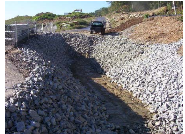
Rock to stabilize channel
