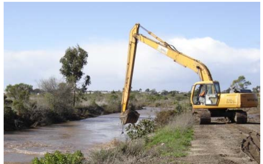
Removing deposited sediment from stream
