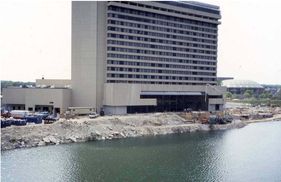
Sediment from construction of motel on Lady Bird Lake
