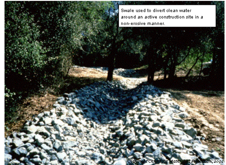
Swale to divert runoff around construction site in non-erosive manner
