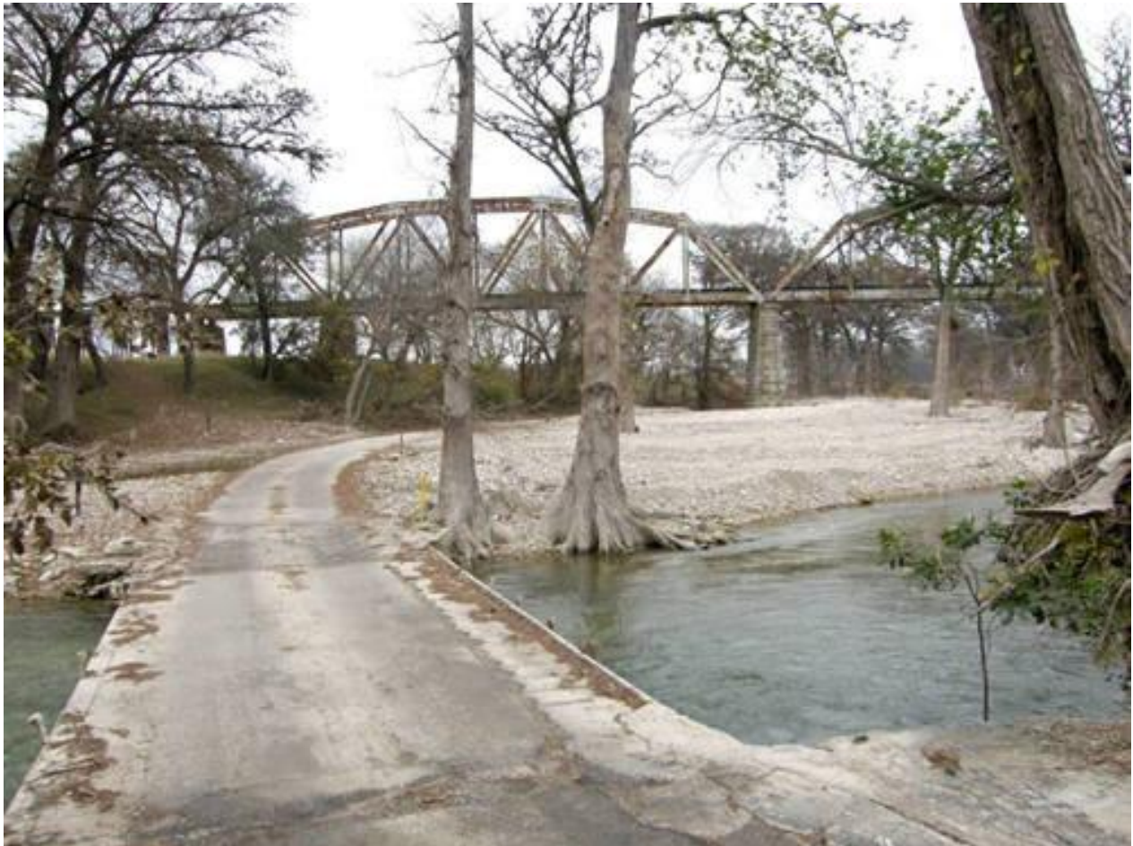
Railroad bridge at Waring (Barclay Gibson)
