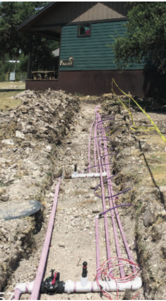
TOP: At Camp Eagle an on-site wastewater irrigation system was substituted for a discharge system keeping pollution out of local waterways.
