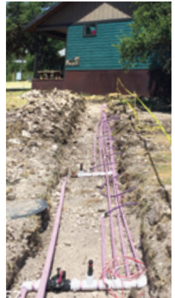
TOP: At Camp Eagle an on-site wastewater irrigation system was substituted for a discharge system keeping pollution out of local waterways.
