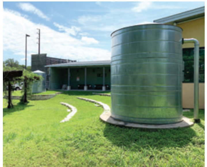
An automated rainwater harvesting system empties in advance of rain forecasts to manage heavy runoff volumes and irrigates the public green space during dry periods.
