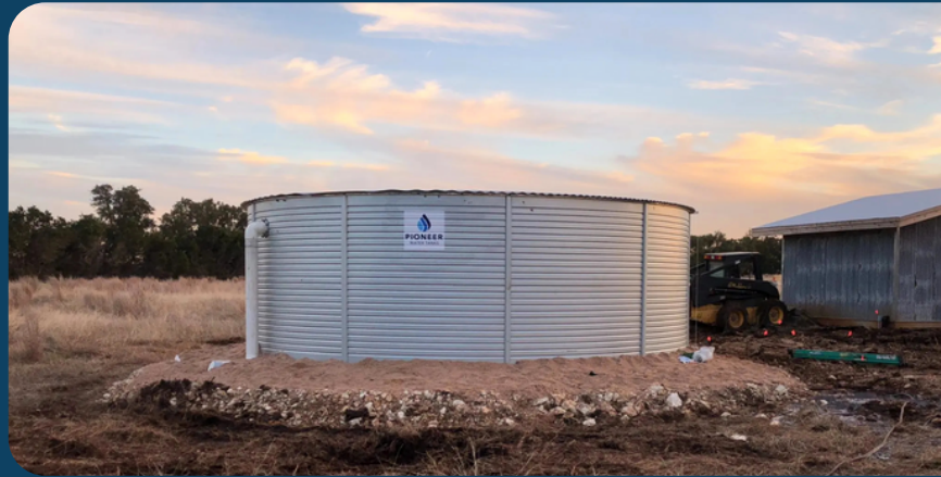
20,000-gallon tank measuring 22' in diameter, 7'2" tall. Minimum recommended for a family of four. Image Source: Harvest Rain
