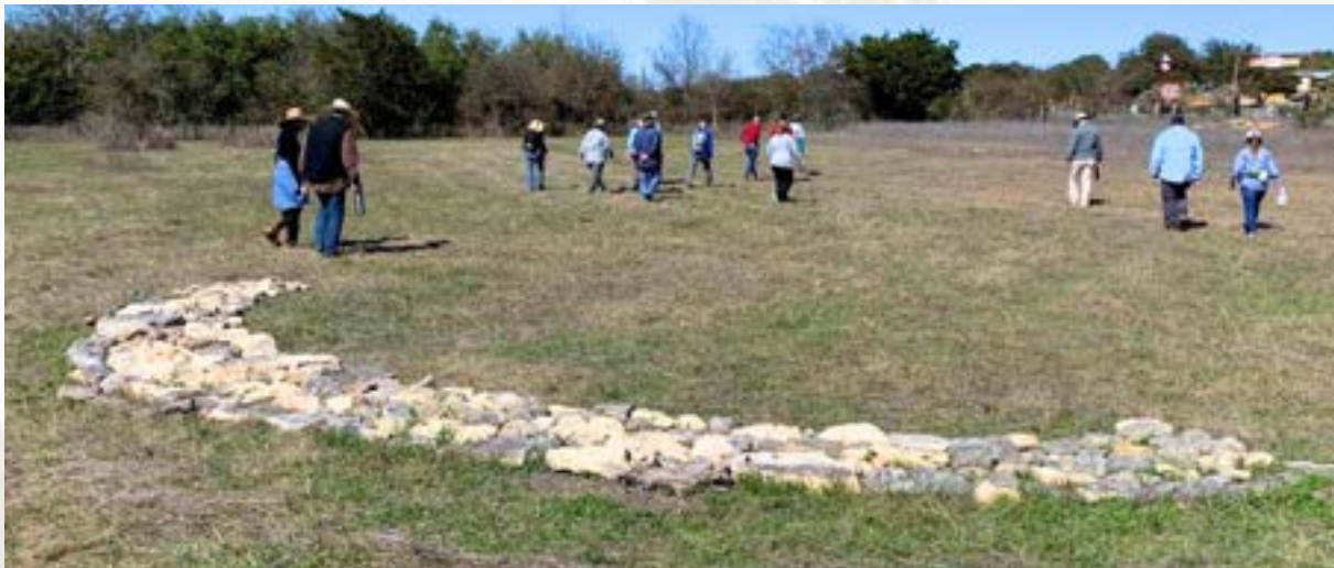
Landowner uses a Media Luna on their hillside to dissipate concentrated water flow
