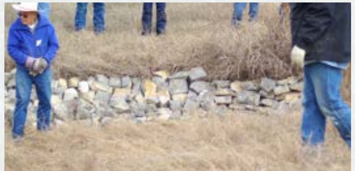
This landowner has used a Rock Run Down to mitigate a low-energy headcut.
