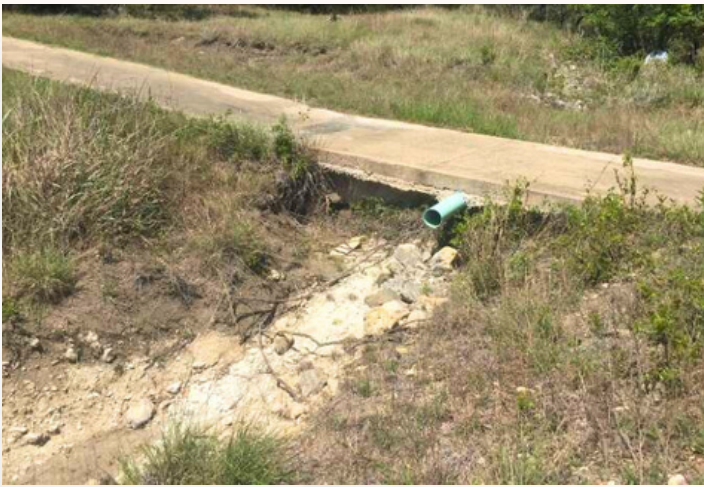
Example of a large headcut that has occurred from an improperly placed culvert
