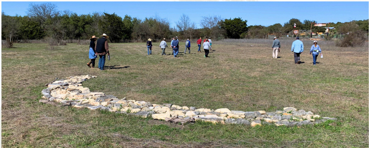
Landowner uses a Media Luna on their hillside to dissipate concentrated water flow
