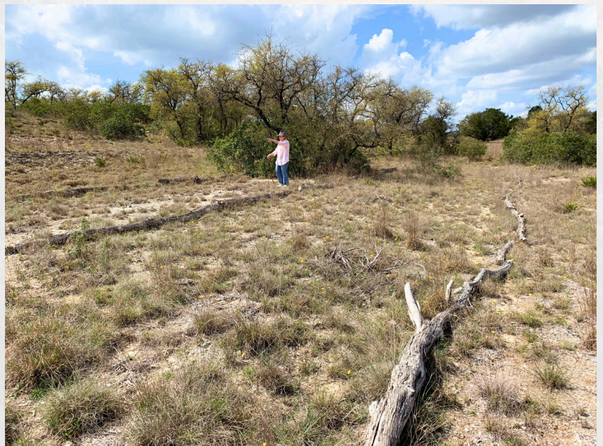
Landowner used three rows of cedar logs to slow and sink water into the land
