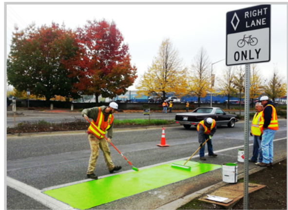
WORKERS PAINTING A BIKE LANE BRIGHT GREEN. PHOTO SOURCE: SEATTLE DEPARTMENT OF TRANSPORTATION
