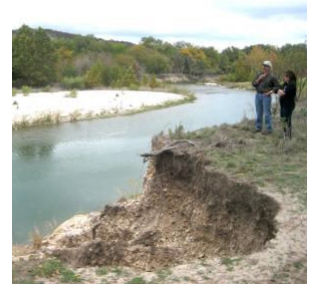
Members of the planning team assess a cutbank and a possible nearby location for the observation tower to overlook the South Llano River.
