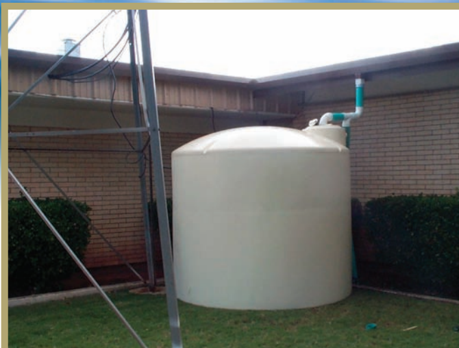
Rainwater Harvesting system at Culberson County Courthouse in Van Horn, Texas
